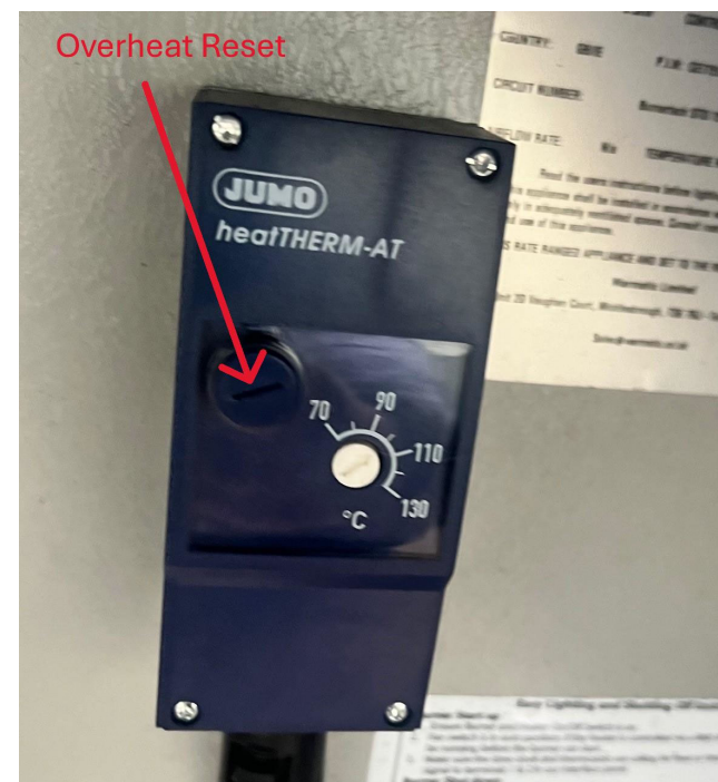
Fig 2, remove the plastic cap with a screw driver and lift the white lever under the cap).
